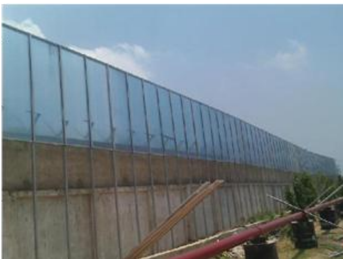
Polycarbonate Noise Barriers incorporated at Zuari Cement by Envirotech
